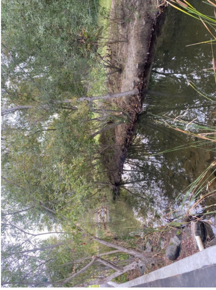
Photograph 5b After. Downed willow tree debris removed. Overgrowth of dead/downed vegetation in understory cleared out. Lower 1/3 of healthy willows trimmed to minimize flow obstructions during flooding events.
